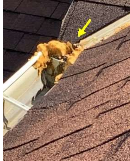
Missing flashing
