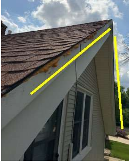
Missing flashing
